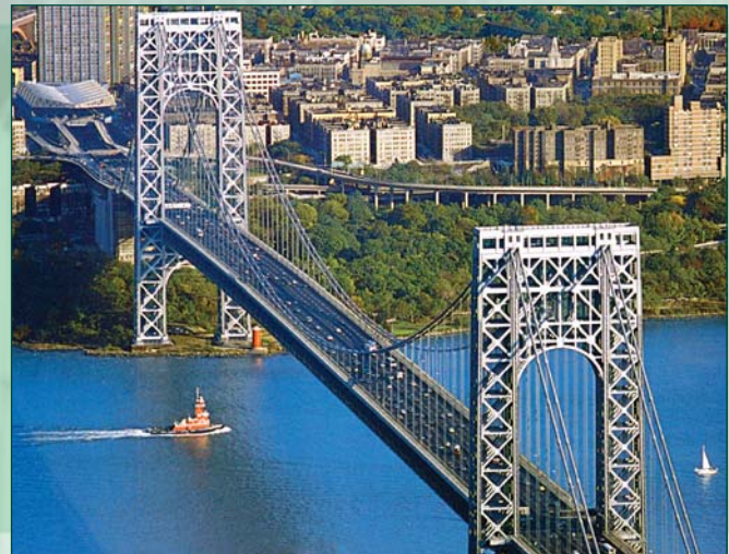
Biennial Inspection & Condition Survey of George Washington Bridge Main Span and NY Approach Spans - PANY/NJ
